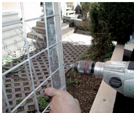
Montage in der Mitte 5-er Loch in Rahmen bohren
